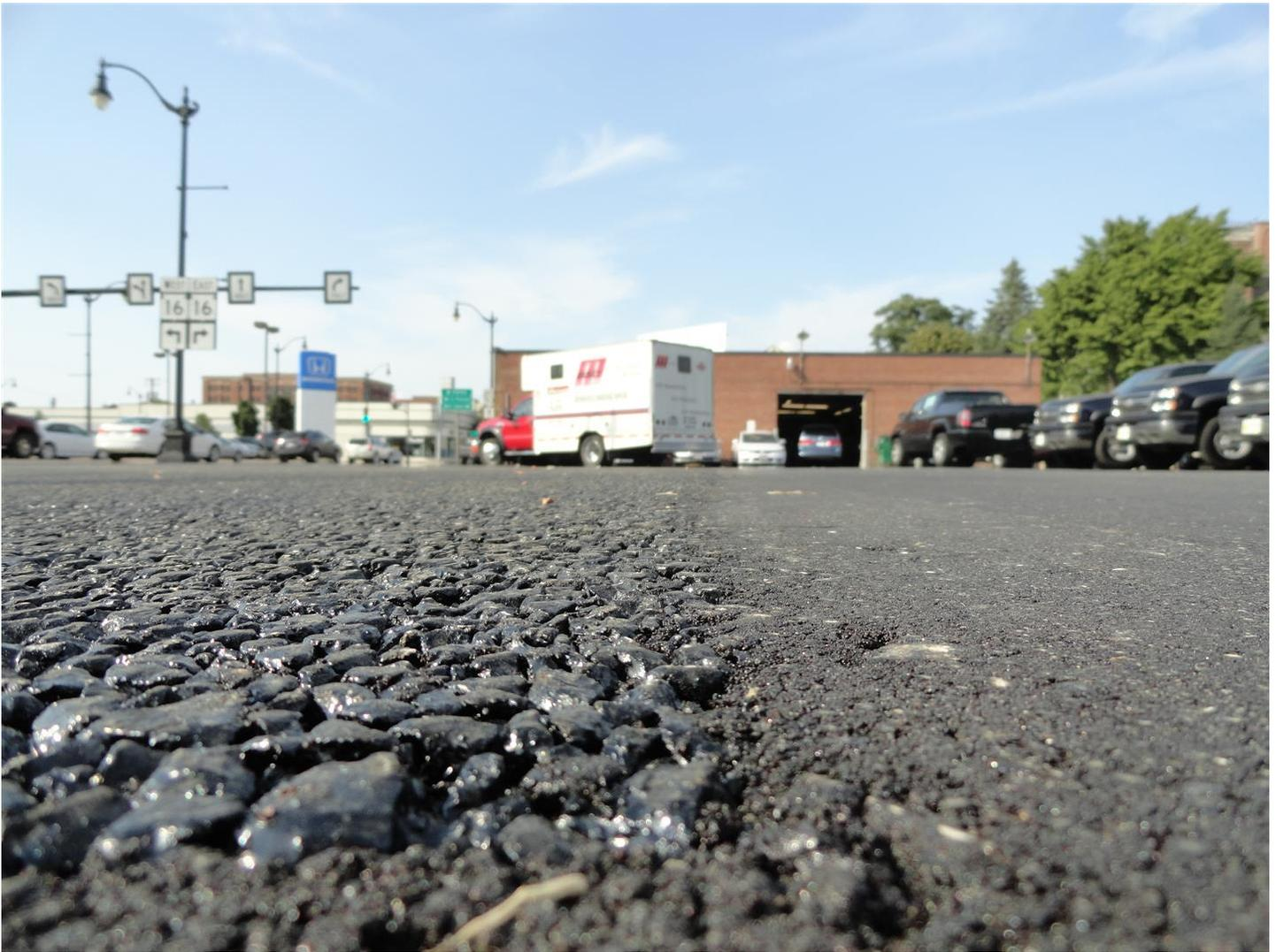
*Honda Motorwerks, in downtown La Crosse, installed pervious asphalt in a portion of their parking lot. Notice the pervious asphalt on the left, and the old, regular asphalt on the right.*
