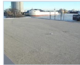
Green roof - before.
