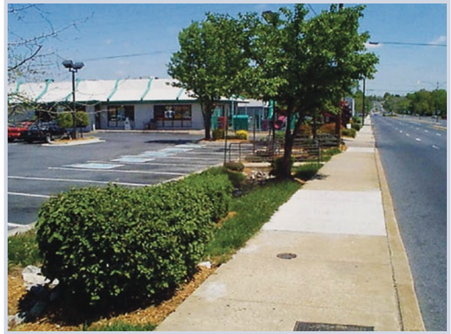
Biofiltration installation.
