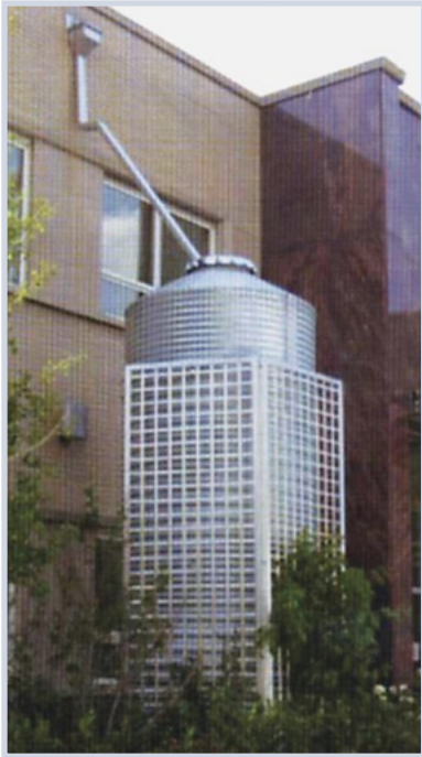
Roof water cistern.
